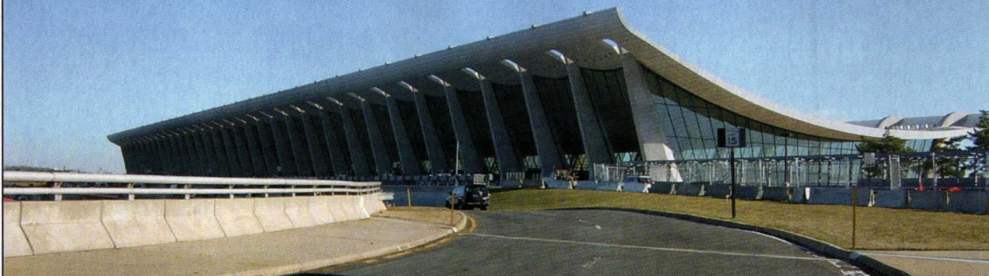
Dulles airport terminal where the terrorists boarded Flight 77
