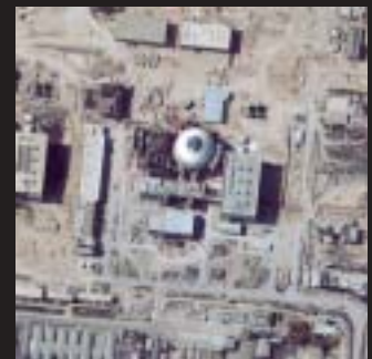
Bushehr nuclear facility - Iran
