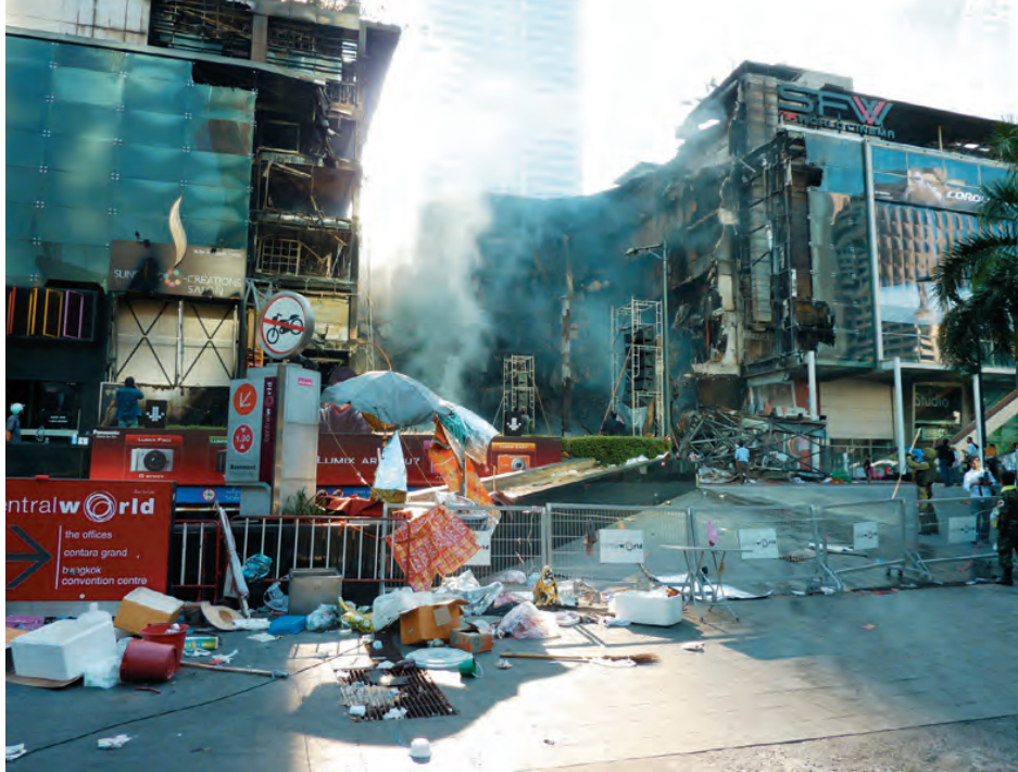
2010. CentralWorld shopping centre in Bangkok following an attack by Red Shirts
