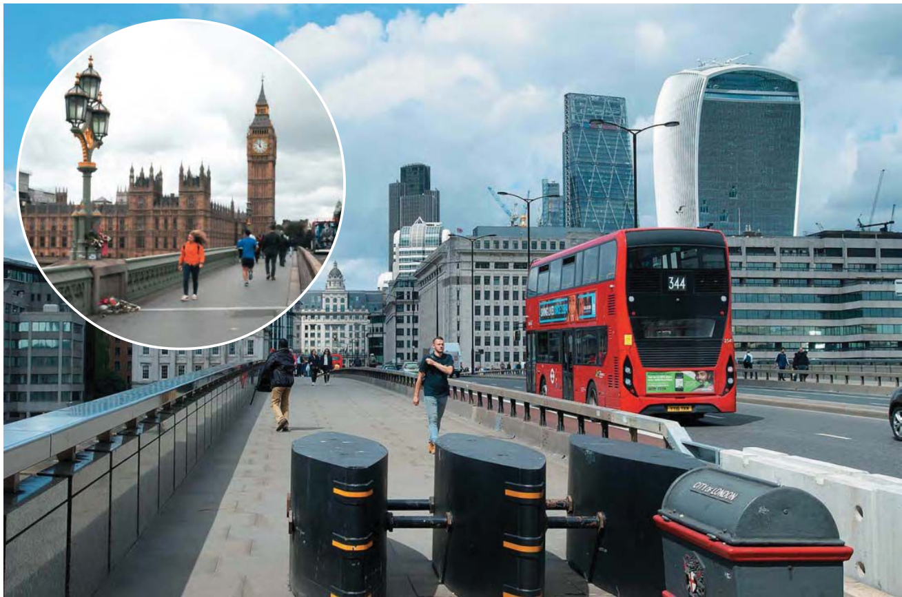
Security piles have now been built on London and Westminster Bridges (inset) to stop vehicles driving on paths. There has been some debate in recent times concerning such structures, but they are set to become part of the 'London scenery'
