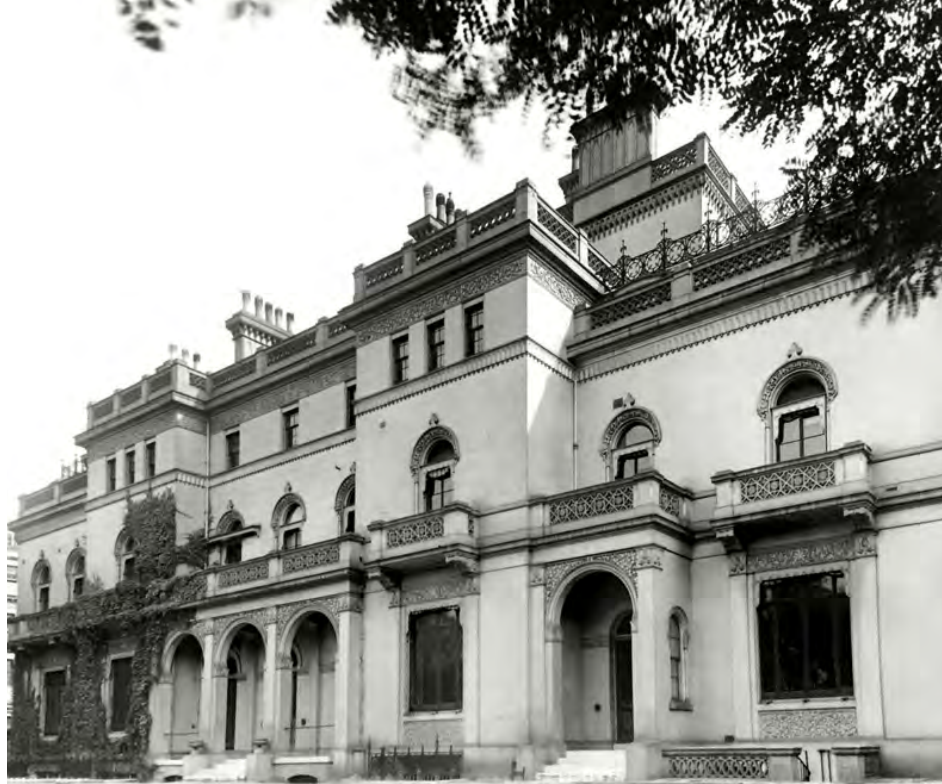
8 and 8a Kensington Palace Gardens 1938. The photograph was taken by the German Section of Britain's Foreign Office as they sought premises for 'special purposes' in the event of war
