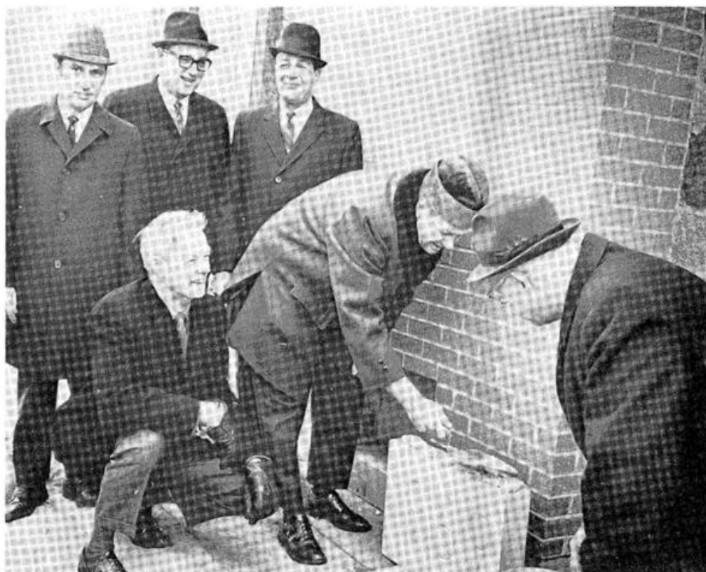
Mayor Tilleman and Chief Madson laying cornerstone
