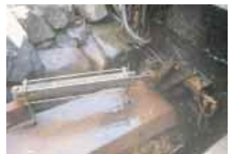
Right: A hydraulic ram, driven by water pressure from the tank 100 meters higher, actuates the butterfly valve.
