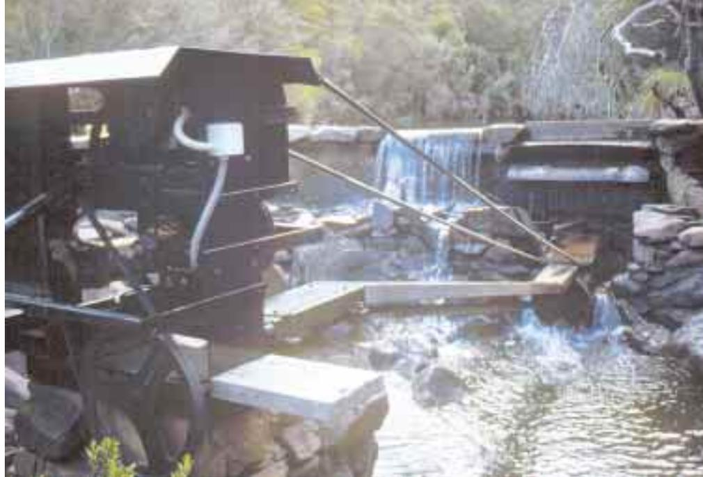
Above: An upstream view of the hydro installation and the 1.2 meter high weir. The "power tower" in the foreground houses the alternator and pump.
