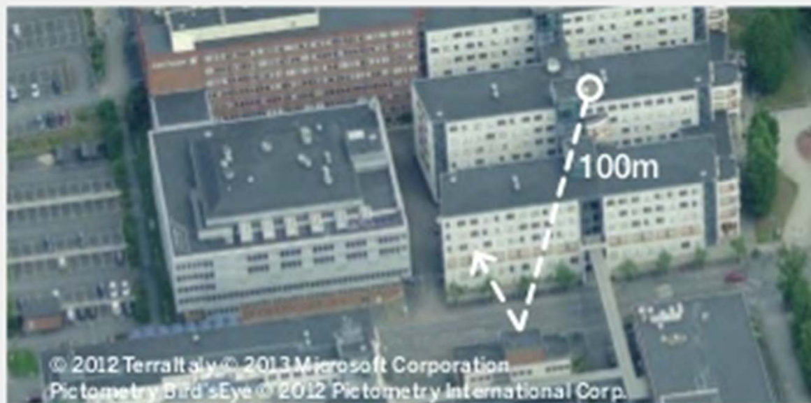
FIGURE 4A Test site for NLOS backhaul - reflection
