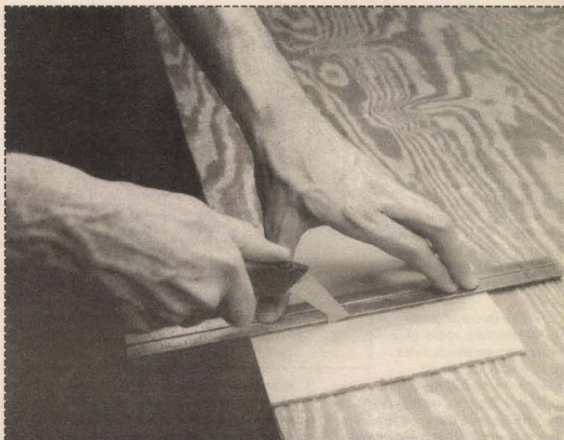
Figure 5. Mark the pieces with a square and a pencil, then use a straight edge and scoring tool to make a groove one-half the material's thickness.
