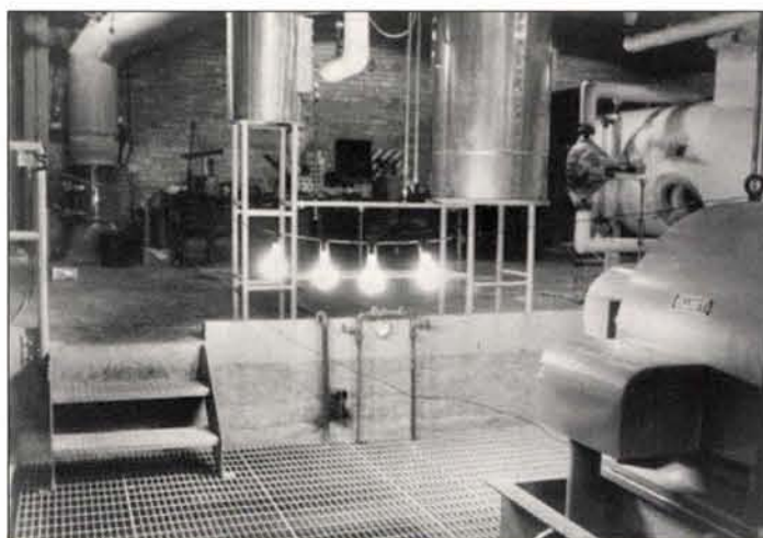
On Dec. 20, 1951, EBR-I lighted four bulbs with the world's first usable nuclear electrical power.
