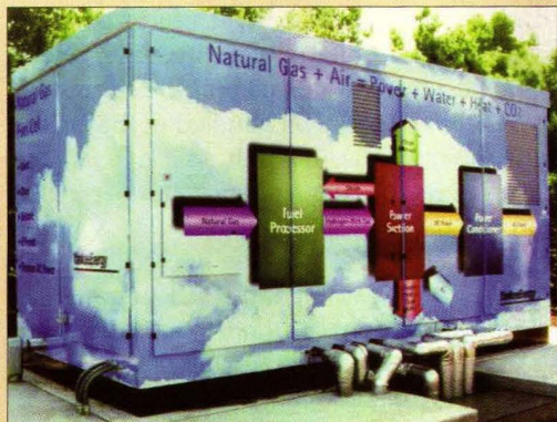
One of UTC's PC25 200-kilowatt power stacking. The graphic on the front of the power plant shows how it works.
