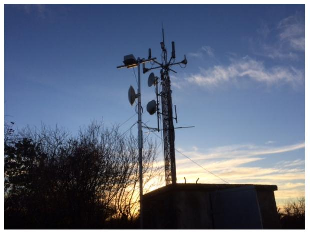
Bell Hill with the new 47GHz beacon on the pole in the foreground (the box at the top of the pole).
