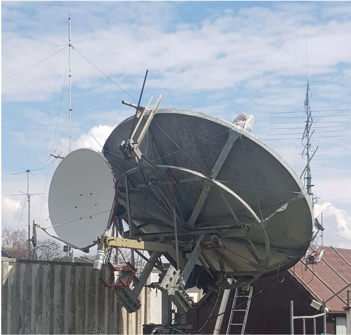
Picture shows the small 1.8m dish mounted at 180 degrees offset to the Large, 3.65m prime focus dish. The feed and associated waveguides have been transferred back to the large dish in this photo.
