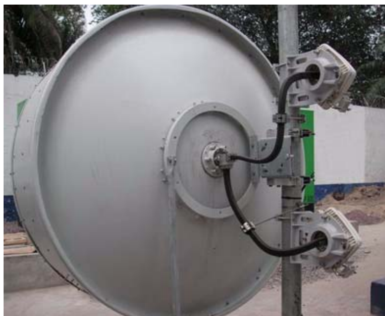
Figure 2-14. Dual Polarized Antenna with Remote-Mounted ODUs
