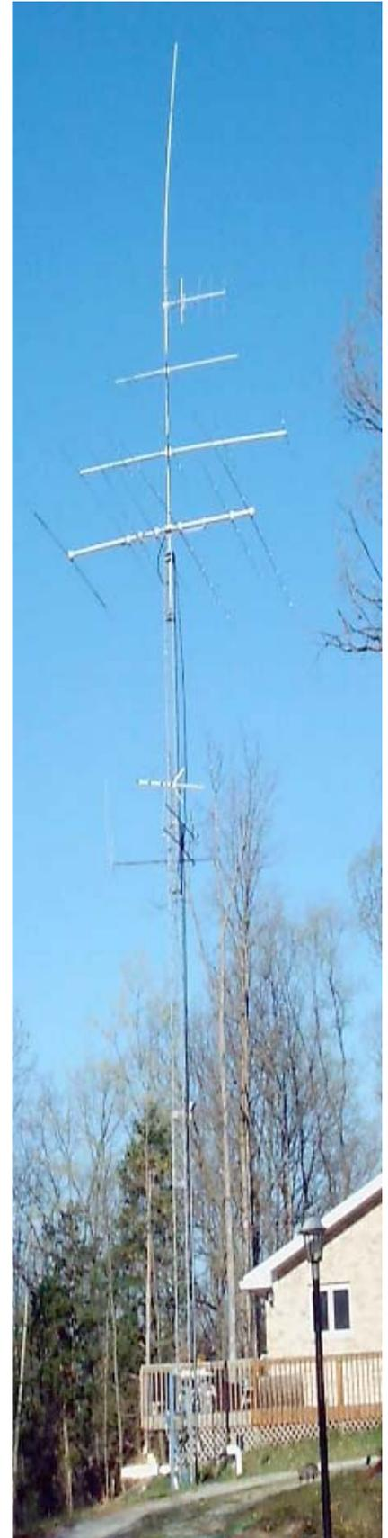
beam antennas at the top of the tower are turned by a Yaesu G-800S rotator.
