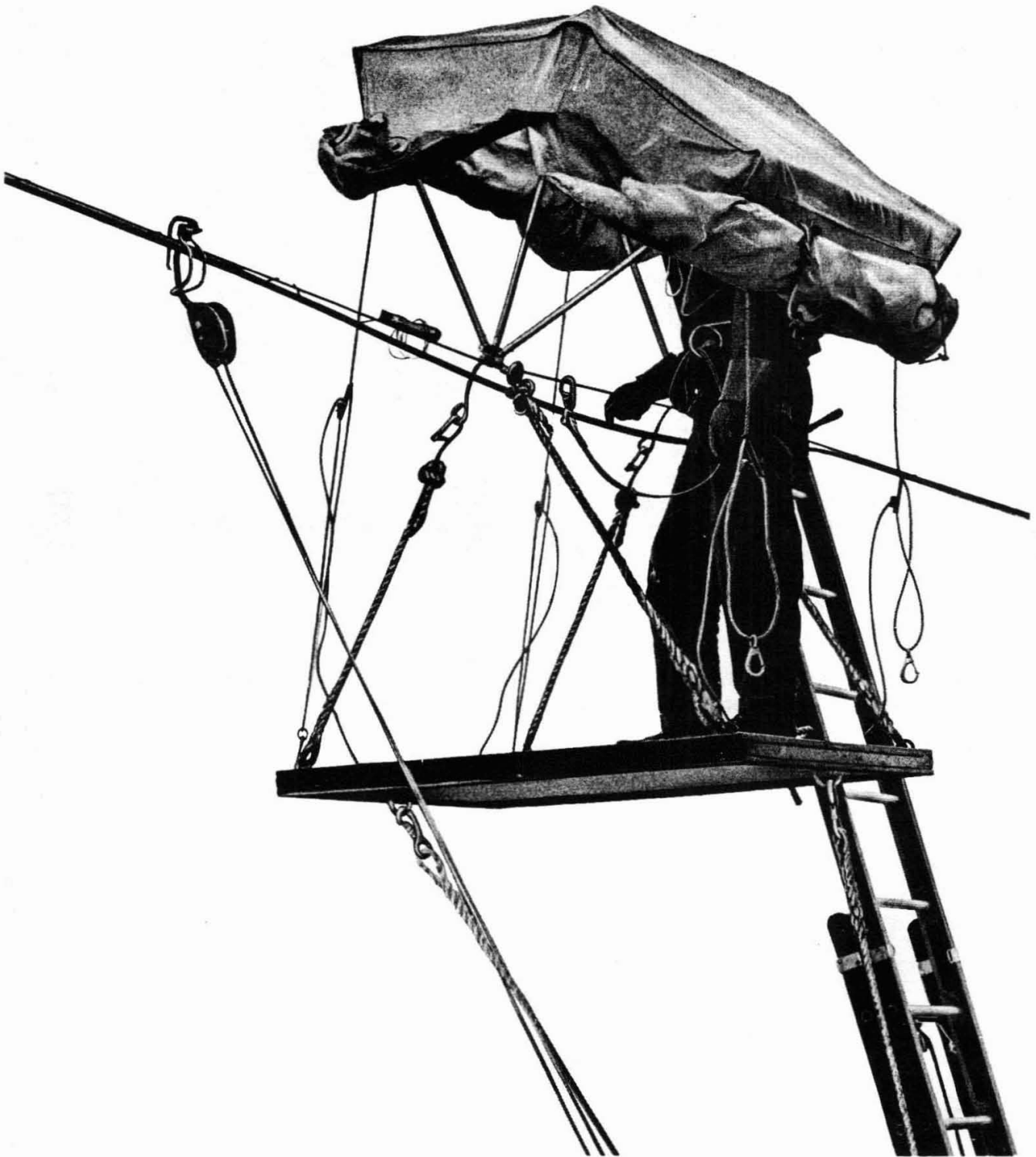
Fig. 7—Platform Placing of Tent—Partially Completed
