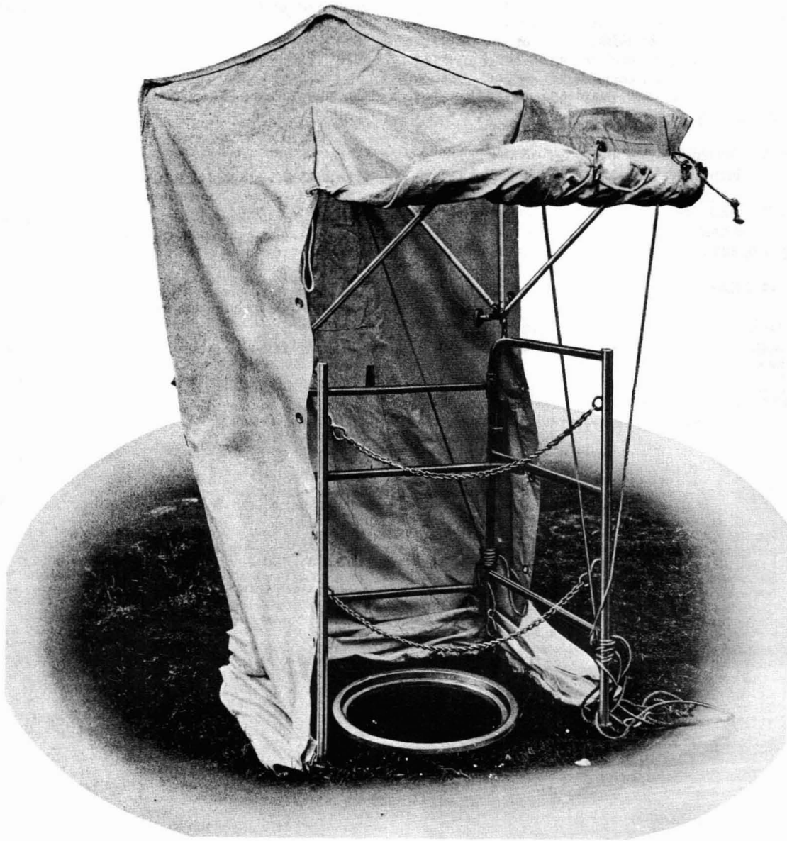
Fig. 11—D Workman's Tent Placed on Manhole Guard
